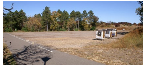
↑ Paved shooting line. BUNKER HILLS ARCHERY COMPLEX , Anoka County, Minn.
